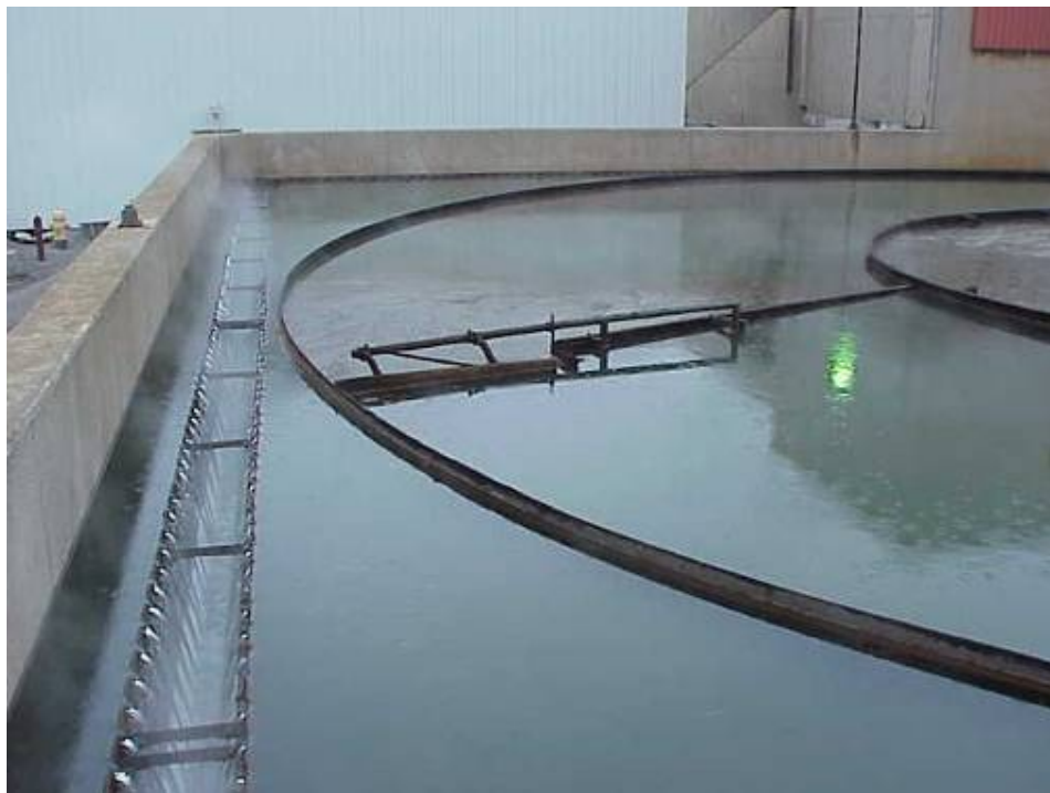
Sludge Thickener
