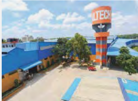
ALTECH ALUMINIUM INDUSTRIES LTD. ETP (Capacity 720 m 3 /day) WTP (Capacity 240 m 3 /day)
